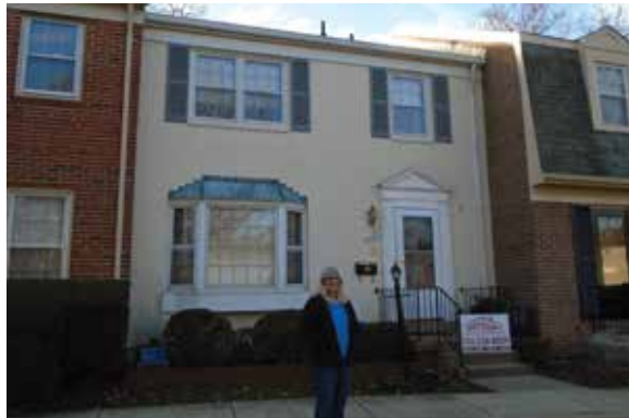
Shari Ashley Blackburn received a new roof system from DryHome Roofing and Siding Inc. through its Free Roof for the Holidays program.
